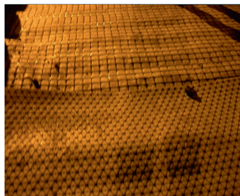
Figure 4.2.3-4: Two kinds of geocomposites after installation
