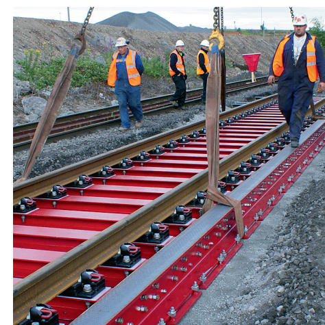
Figure 4.3.1-1: Pre-assembled panel lowered onto the formation
