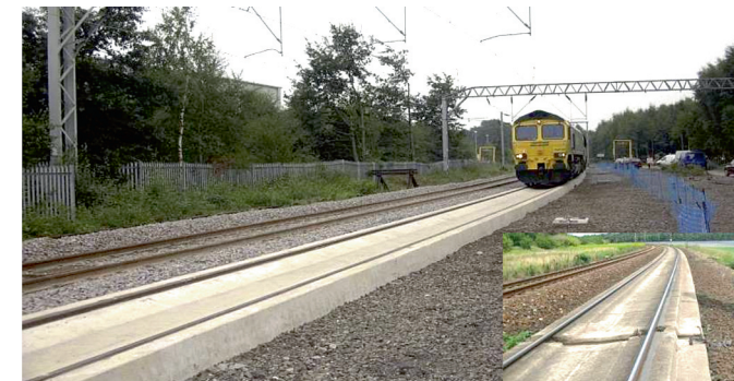
Figure 4.3.2-1: UK installation of BB ERS system (Waghäusel site)
