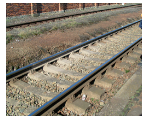
Figure 4.2.3-2: Station track with clear drainage defects
