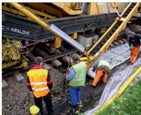
Figure 4.2.3-3: Old ballast removal with geocomposite installation
