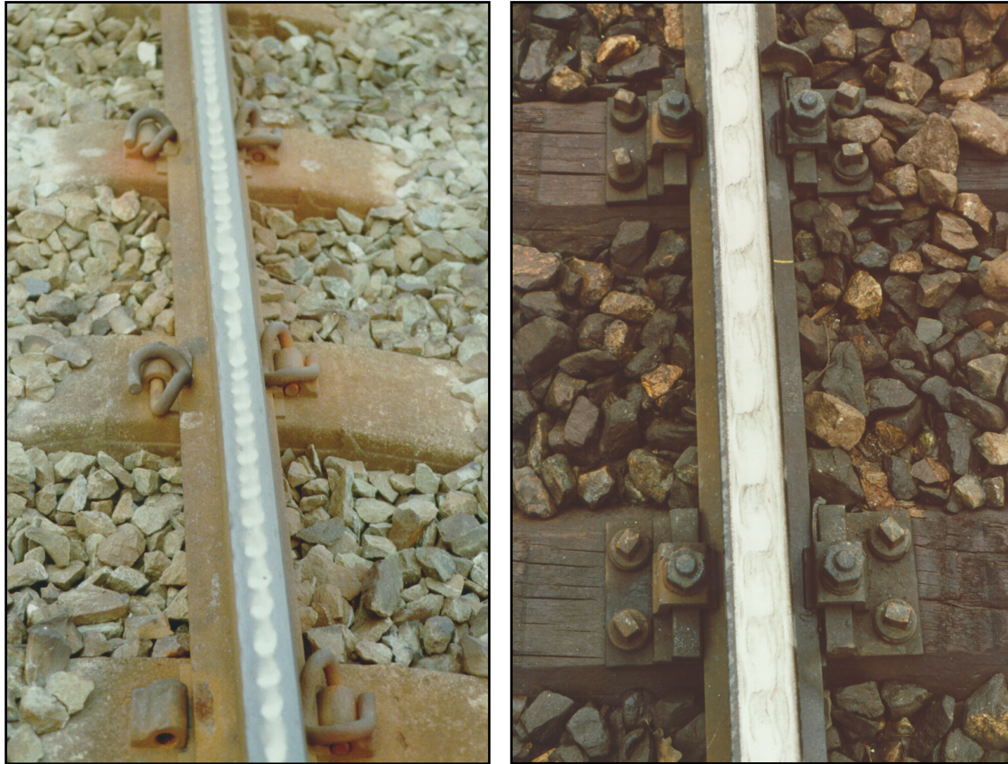
Figure 4-1: Short pitch corrugation (left) and short wave formation (right)
