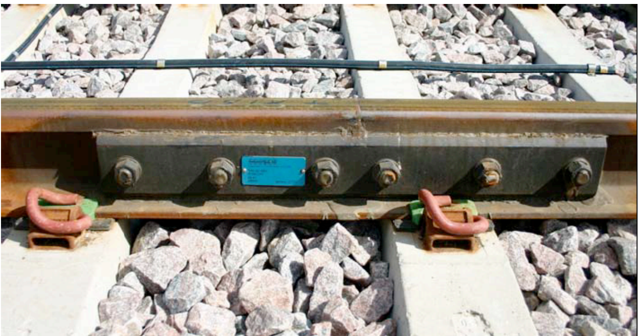
Figure 1 A newly installed insulated joint on The West Coast Line in Sweden
