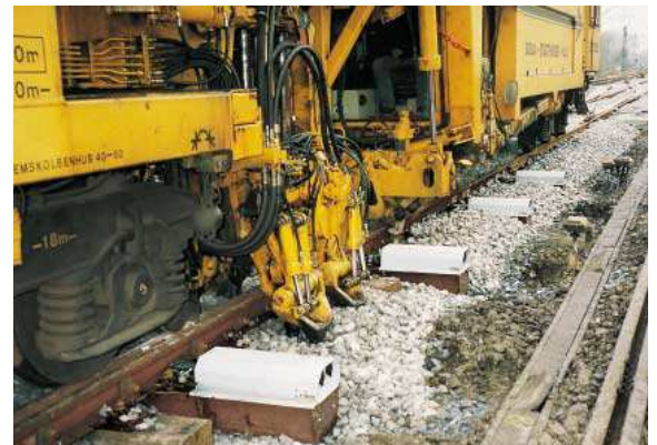
Figure 7: Machined tamping of a switch equipped with multiple actuators
