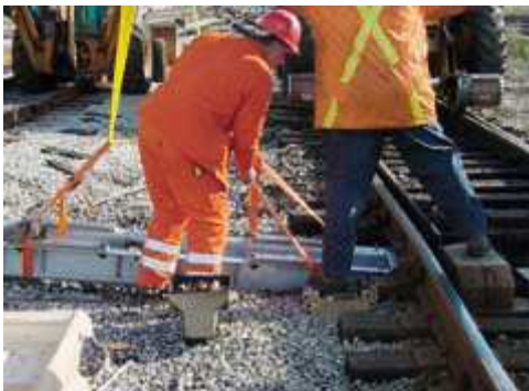
Figure 6: Installation of a hollow sleeper drive into a already installed switch (6)
