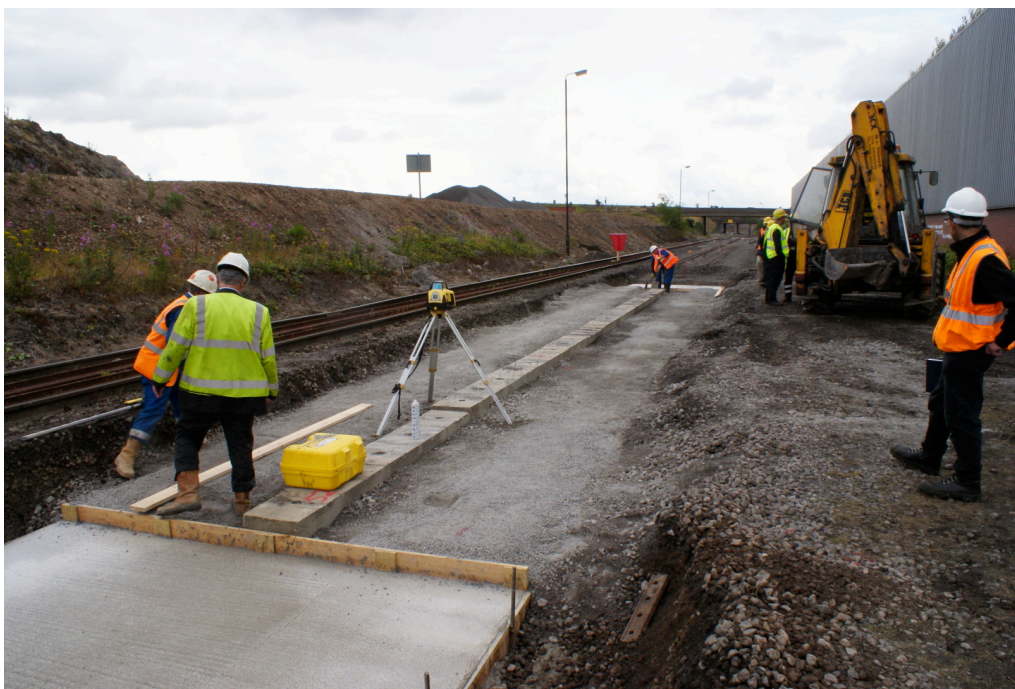
Figure 5 Central spine of support blocks. This can also be a steel beam with intermediate screw jacks. In the foreground is the concrete base for a transition.
