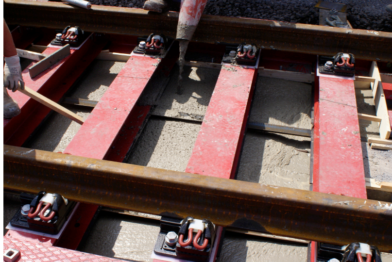
Figure 8 Concrete pour to form base during a later possession after track has been opened to traffic.
