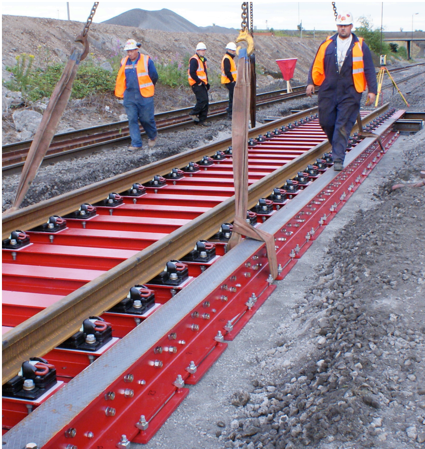
Figure 3 Pre-assembled panel lowered onto formation
