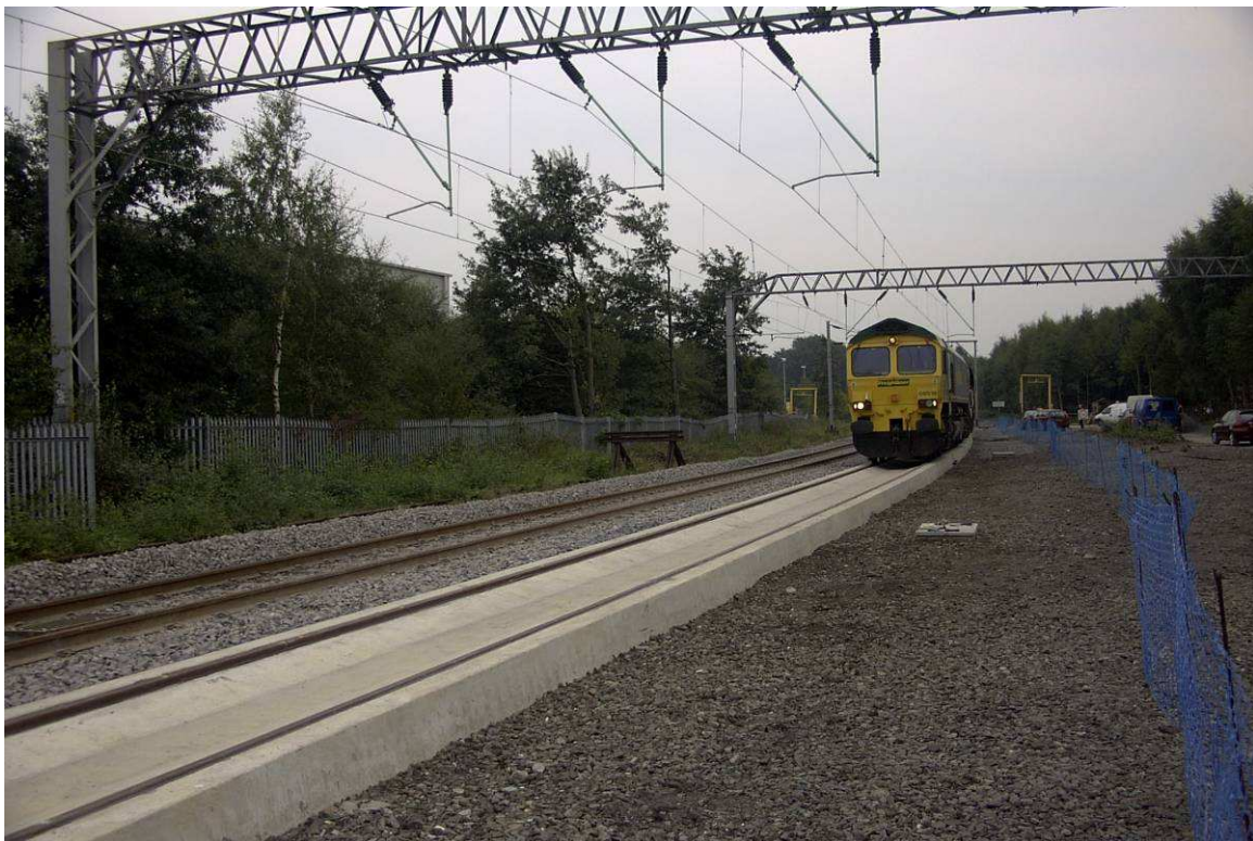
Figure 3.1-1 Mkl BB ERS trial length installed on West Coast Main Line in Crewe, UK
