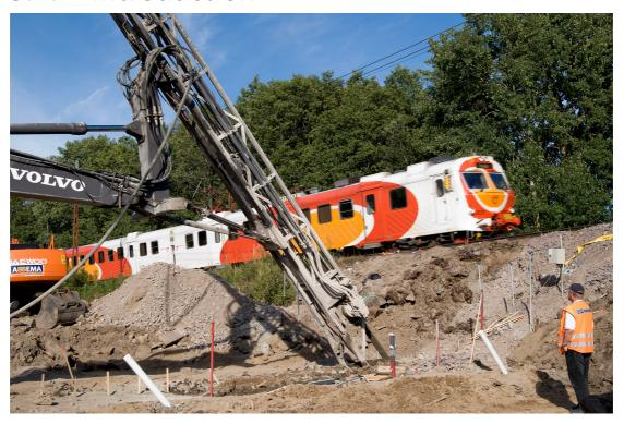
Installation of subgrade strengthening under an existing track and undergoing railway operation is a demanding action. Requirement for comprehensive preparation is obvious and there are many steps that have to be done very carefully and in advance. The following guideline gives an overview of issues that are important to pay attention to:
