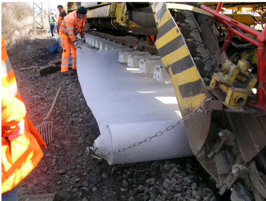
Fig. 5: Placement below ballast
