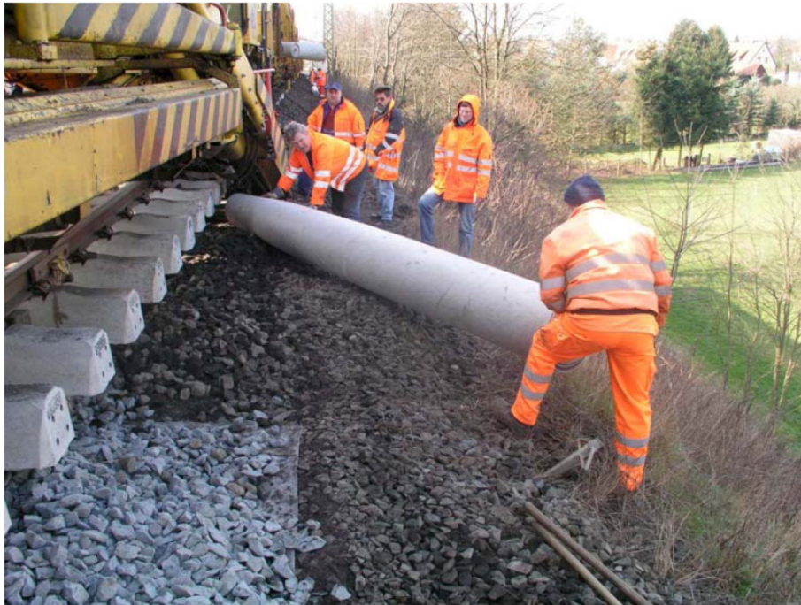
Fig. 4: Preparation of geotextile roll
