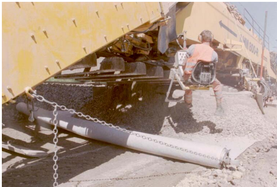
Fig. 7: Geotextile is fixed on the maintenance machinery
