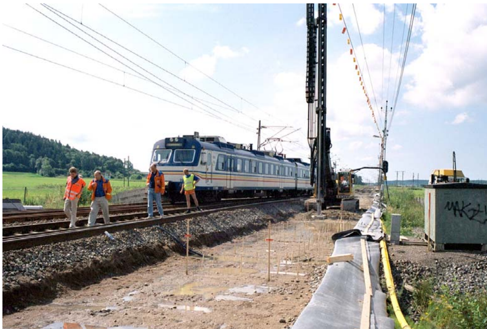
Installation of lime-cement columns (Ledsgård /Sweden July 2000)
