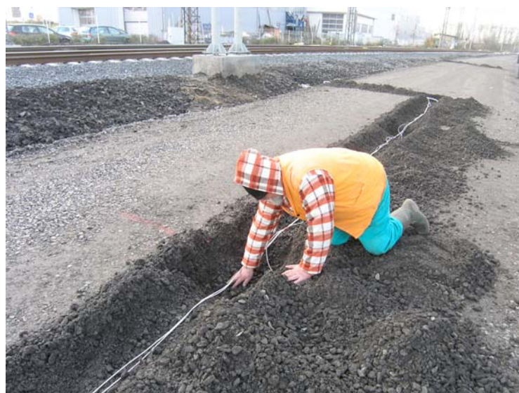
Fig. 8: Building up the seismic monitoring base at Běchovice site in the time of track reconstruction
