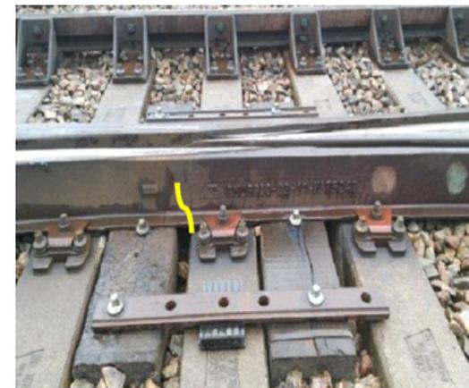
Figure 65-1 Common crossing cracked in the foot flange area (crack in yellow)
