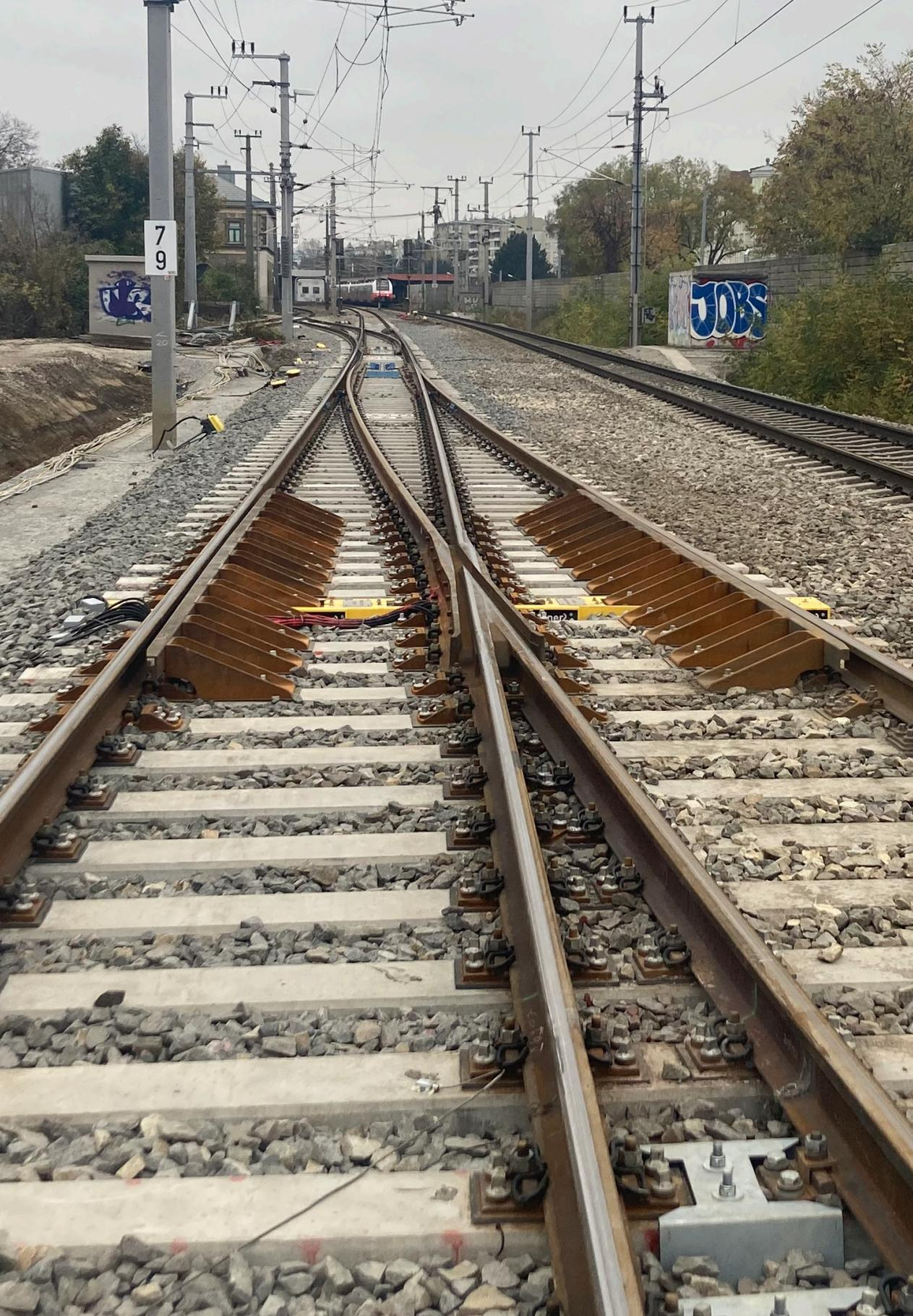
optimised nominal stiffness of 25 kN/mm in the frog area and 60 kN/mm in the check rail plate area. By adjusting the intermediate plate stiffness beneath the frog area alone, a 10% reduction in static ballast pressure was achieved. This additional elastic layer was matched to the polyurethane under sleeper pads which are already a standard for turnouts at ÖBB.
