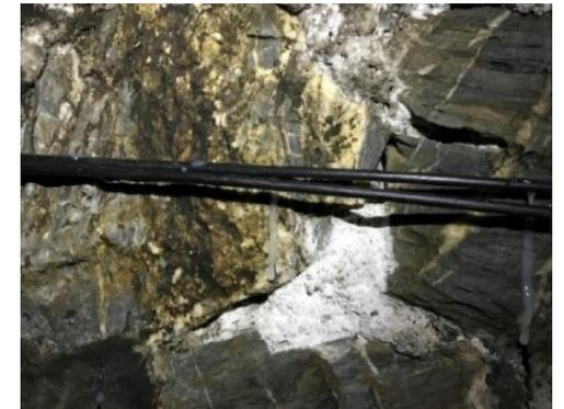
Figure 55-2 Fixation with facing irregularity
