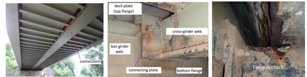
**Figure 75-1** Detail of connection susceptible to fatigue cracking
