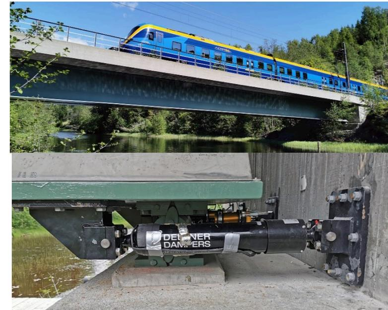
Figure 68-1 Top: view of the bridge during passage of an X62 train, bottom: details of the retrofitted damper near the roller support.
