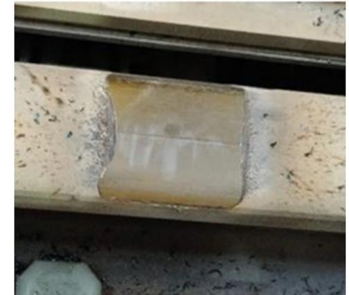
Trials have been carried out to extend the sections and grades that can be repaired. Rail grades R200, R220, R260 in 56E1, 60E2 and similar predecessor sections have been repaired. HP335 grade has been repaired and metallurgical results are excellent.
