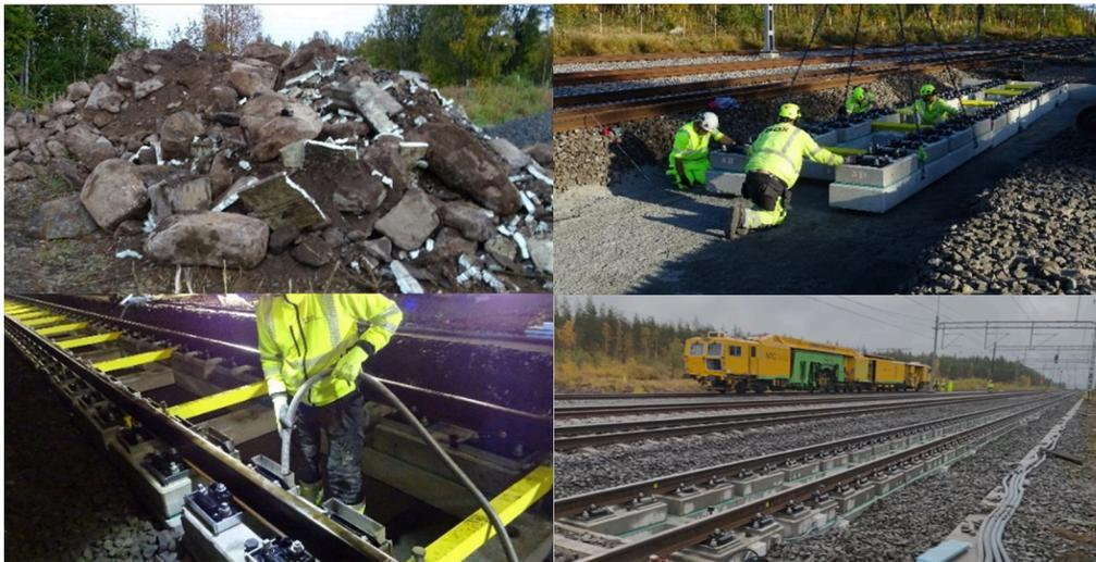
Figure 62-3 Large boulders found during excavation (upper left), whole modules being positioned (upper right), pouring of levelling mortar (bottom left), finished track section at 96 hours (bottom right).
