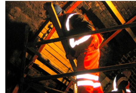
Figure 74-1 Traditional method of undertaking tunnel brickwork repairs
