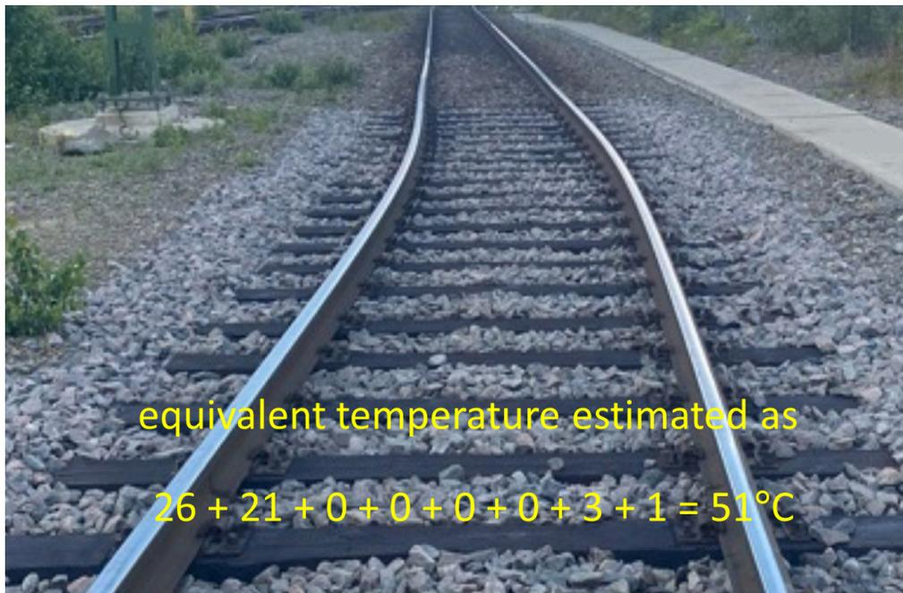
Figure 24-1 Track buckle with corresponding evaluation of equivalent temperature as a sum of contributing factors. Picture Trafikverket.
