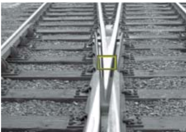
Crossing nose and its finite element modelling in project MU14 (see drawing of switch on page 21)
