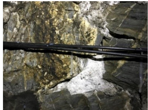
Figure 55-2 Fixation with facing irregularity
