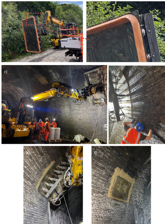
Figure 74-2 The flexible plate for the demonstrator (a), detail of perimeter seal, (b) execution of the repair (c, d and e) and patch repair after removing flexible plate
