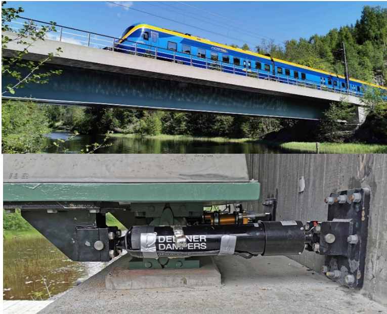
Figure 68-1 Top: view of the bridge during passage of an X62 train, bottom: details of the retrofitted damper near the roller support.
