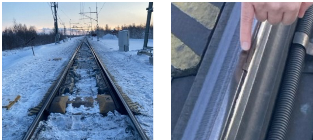
Figure 30-1 Left: Switch & crossing at the Iron Ore line. Right: Plastic deformation of the tip of the switch rail.
