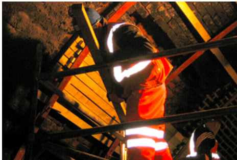
Figure 74-1 Traditional method of undertaking tunnel brickwork repairs
