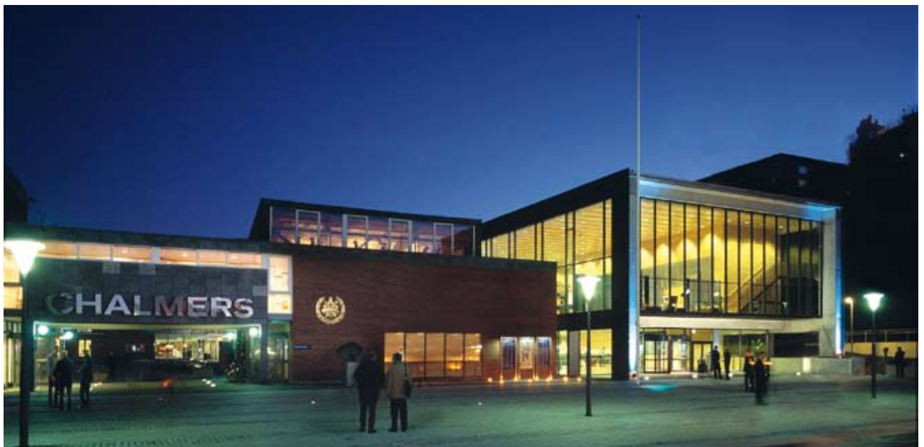
Main entrance to Chalmers University of Technology with the Student Union building on the right
