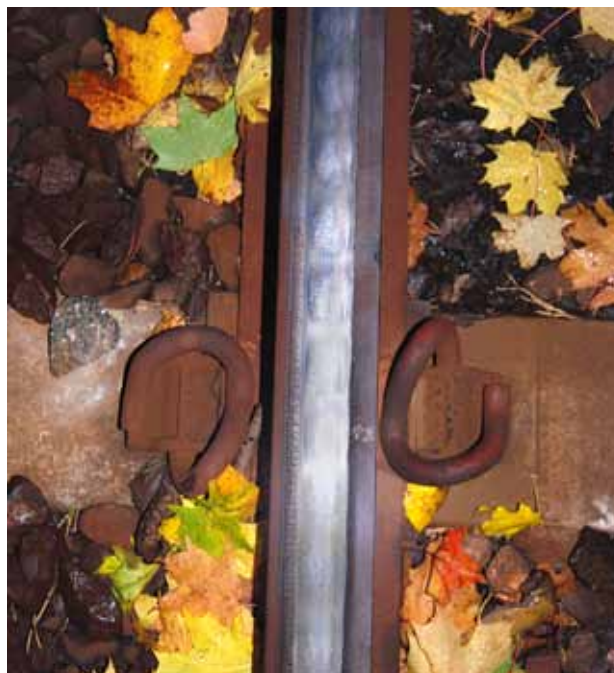
Corrugation of low rail on a curve of SL track at Stora Mossen in Stockholm
