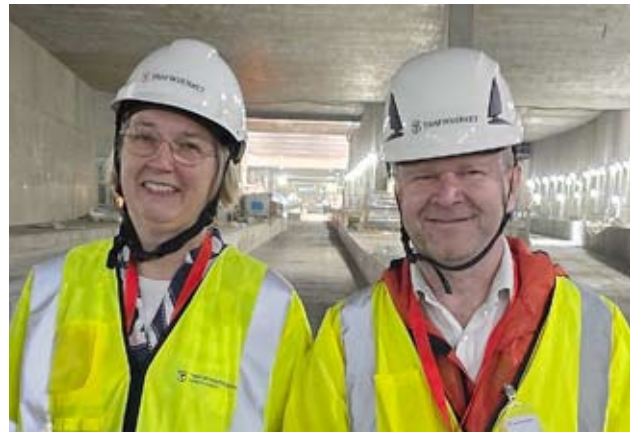
Pernilla Edlund from Trafikverket and Anders Ekberg in the tunnel leading to the new underground West Link station at Gothenburg Central Station
