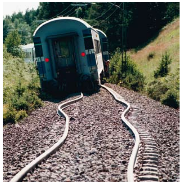
Derailement of the last two coaches in a Swedish passenger train on 6 July 1997 between Låstringe and Tystberga on a regional line south of Stockholm and north of Nyköping. The day was calm with few clouds and a maximum temperature of about 25 °C. According to eyewitnesses, the lateral buckling and displacement of the track gradually increased as the train braked
