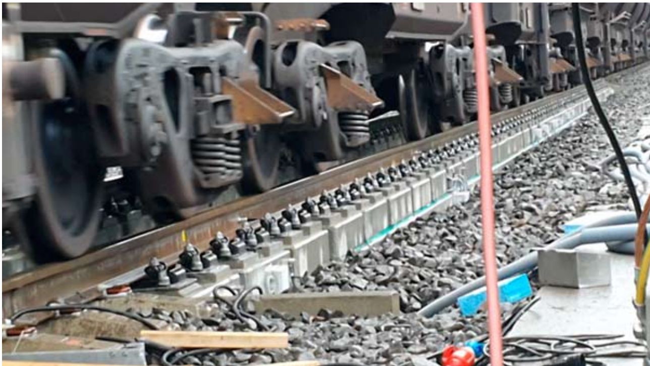
Iron ore train passing the instrumented transition zone between ballasted track and 3MB slab track at Gransjö in project TS22 (image from movie)
